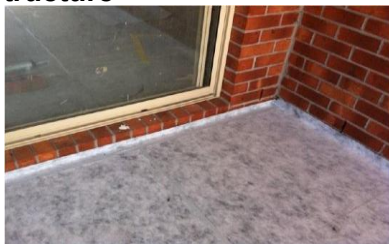
Application of Inoplast PL
